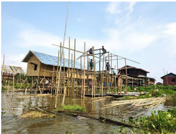
Figure 4-2 Donor’s Funded Stilt House Newly Built in Place of Collapsed One on Lake Water
